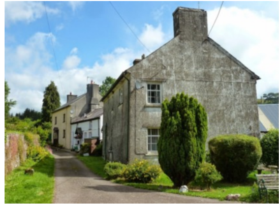
Llywel village and the former Cross Keys Inn (nearest)
