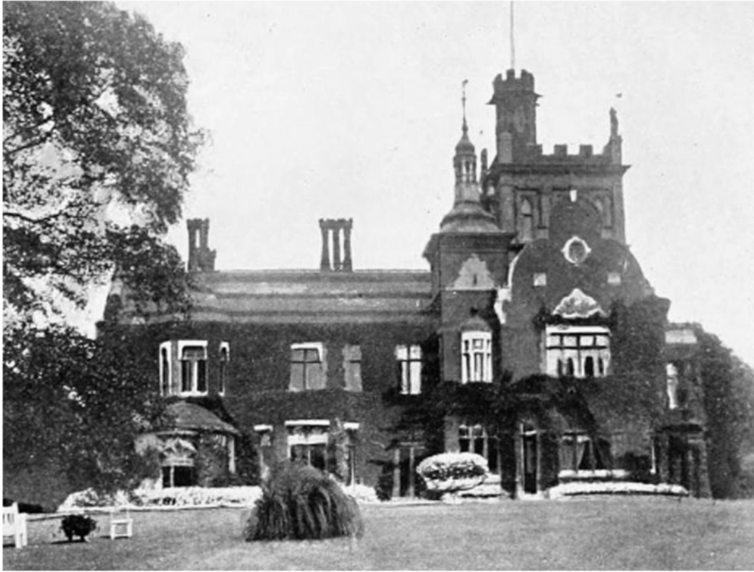
Caen-wood Towers - Highgate
